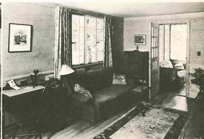
(Above) Painted cinder block for interior walls and the warm browns and reds of the precast floor have proven both economical and satisfactory. (Right) The walls of living room have horizontal pine ship lap below the dado and plywood above
