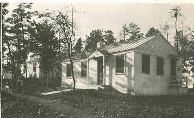
Four-room houses of cinder block (Type A) with paint finish. Floors are concrete slabs and roofs of metal. They are vermin and termite proof and also fire-resisting. Thirty such houses, with numerous exterior variations, were built
