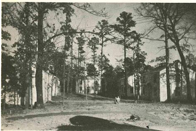
These houses (Types C and D) are built of cinder block with no other finish than paint, both inside and out. Floors are precast concrete slabs on reinforced concrete joists. Heated by coal stoves
