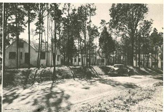
A group of houses on Pine Road including (left) a five-room house (Type 54) and four-room houses (Type 41). A primary consideration was to take advantage of good sites without felling trees
