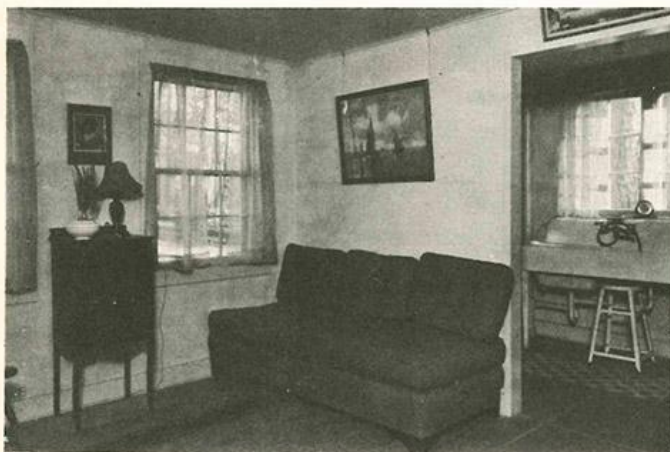
(Above) Painted cinder block for interior walls and the warm browns and reds of the precast floor have proven both economical and satisfactory. (Right) The walls of living room have horizontal pine ship lap below the dado and plywood above
